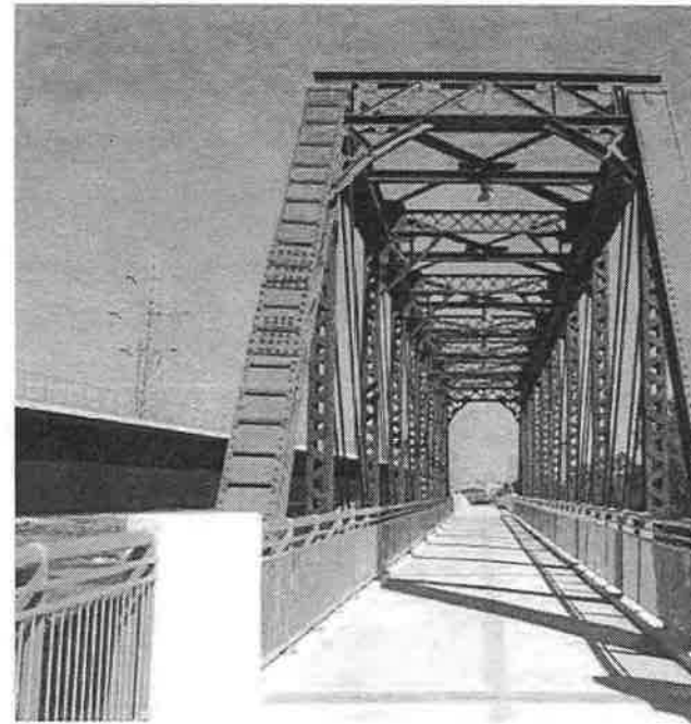
Santa Fe Trestle – Santa Fe, NM
